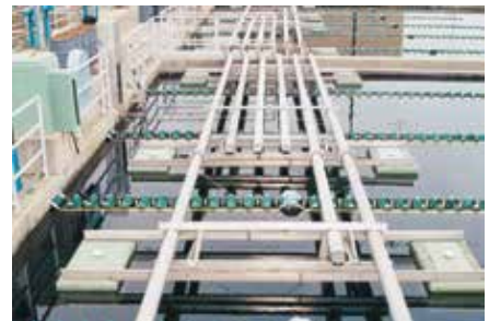
Water & Wastewater Treatment
